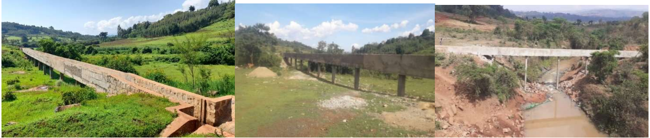
Figure 12: Depressed area and Gibe River Crossing Flume construction completed
