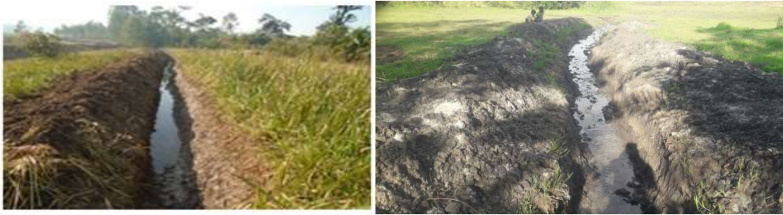
Fig 10: Drainage canals excavated
