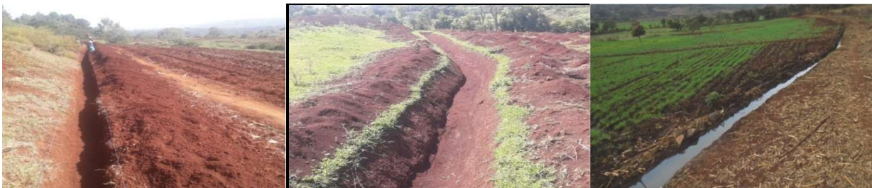
Figure 9: Completed Secondary Canal sections
