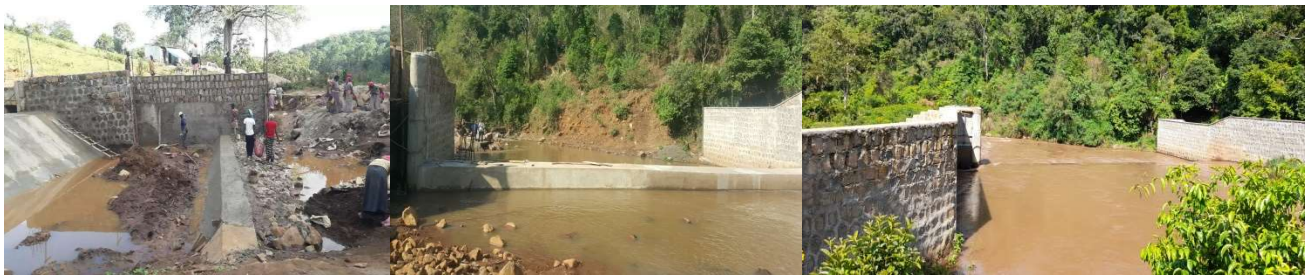
Figure 3: Weir body constructed & completed
