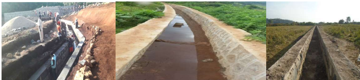
Figure 6: Lined canal constructed
