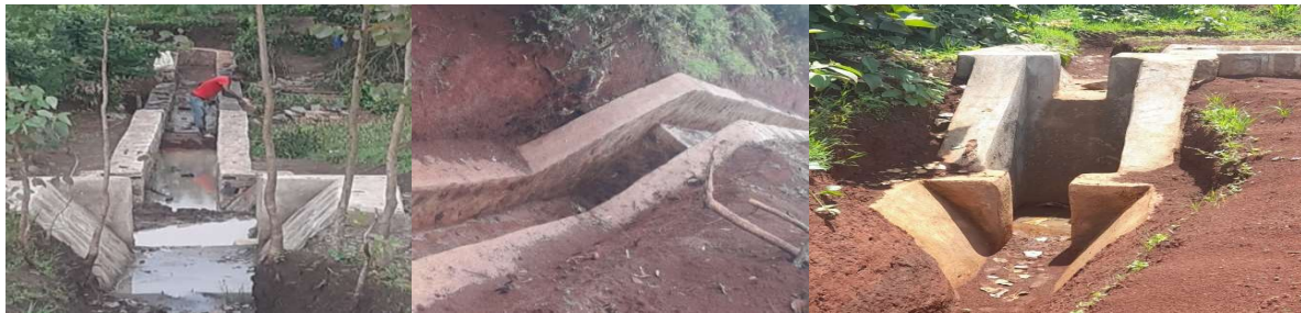
Figure 15: Drop Structures constructed
