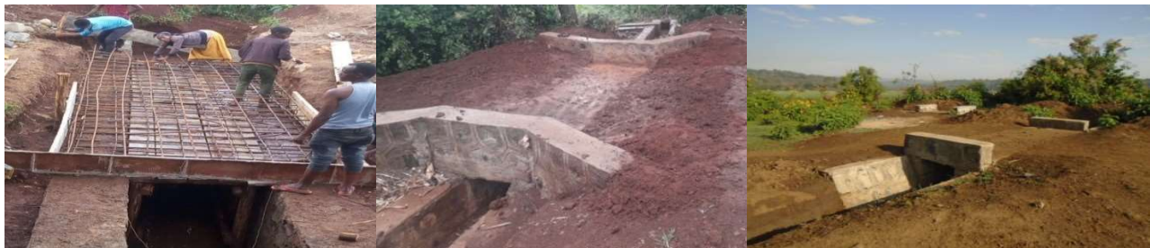
Figure 13: Completed Road culverts
