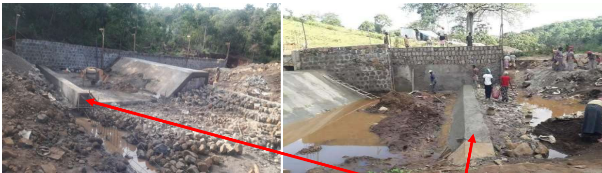
Fig 19: concrete end sill constructed
