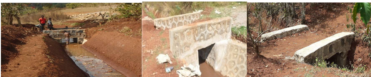
Figure 11: Completed Foot bridges
