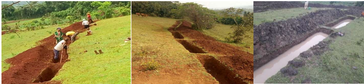
Figure 27: Soil bunds excavated to protect the canal and canal structures
