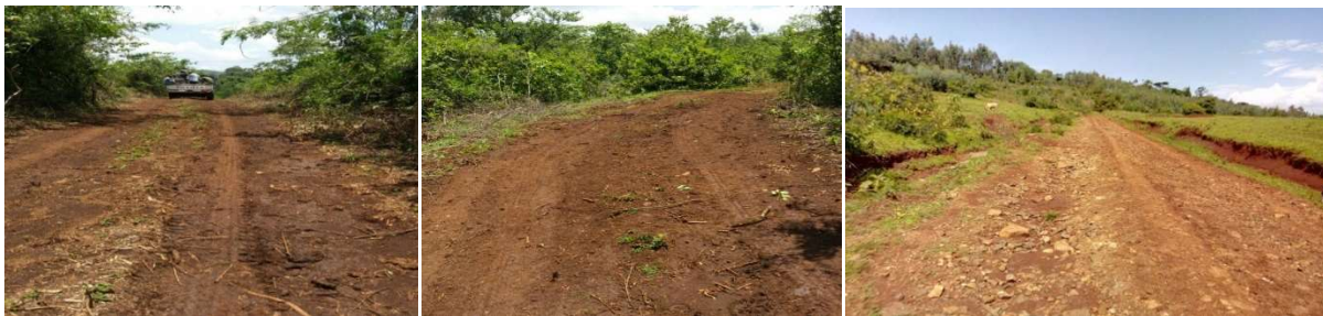
Fig 2: Access road maintained
