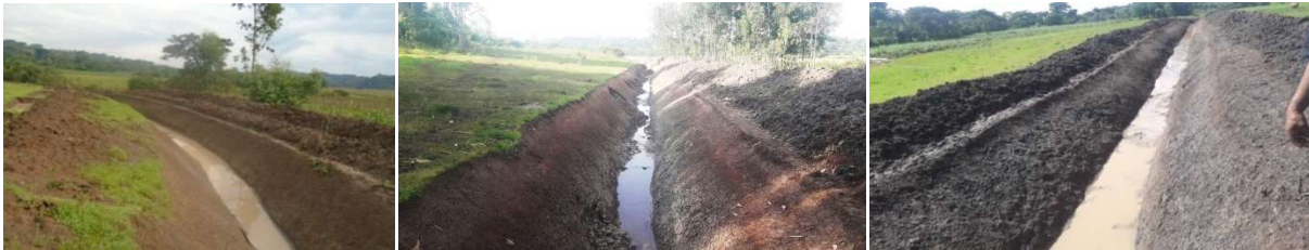
Figure 8: Branch Canals excavated
