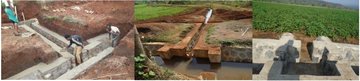
Figure 16: Division boxes constructed on main & Branch Canal
