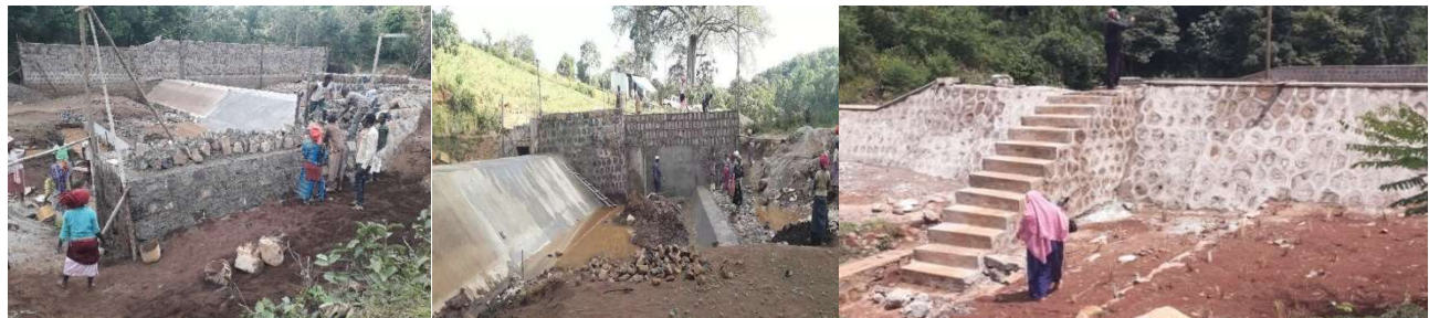
Fig 4: Retaining wall & walking stair completed
