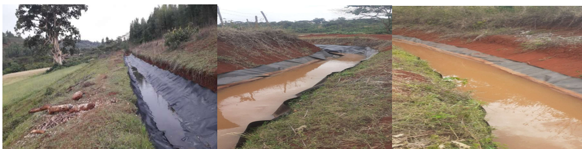
Fig 20: Leakage canal areas protected by covering with Geo-membranes
