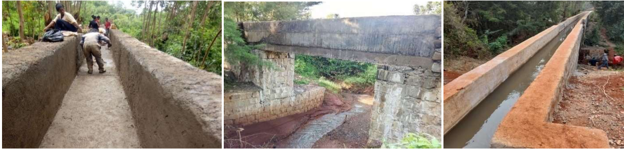
Figure 14: Drainage culvert constructed
