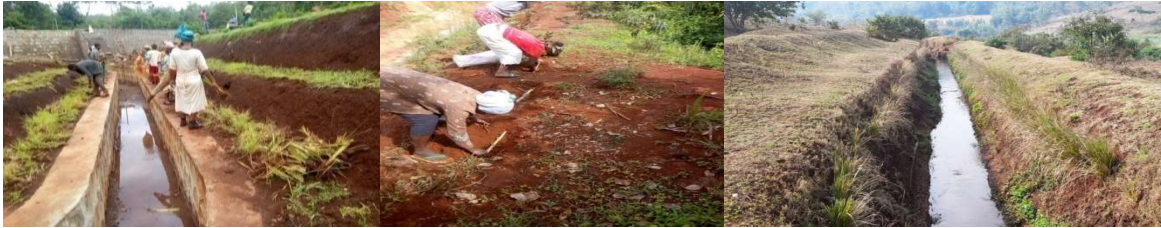
Fig 31: Vetiver planted at the canal and soil bund embankment
